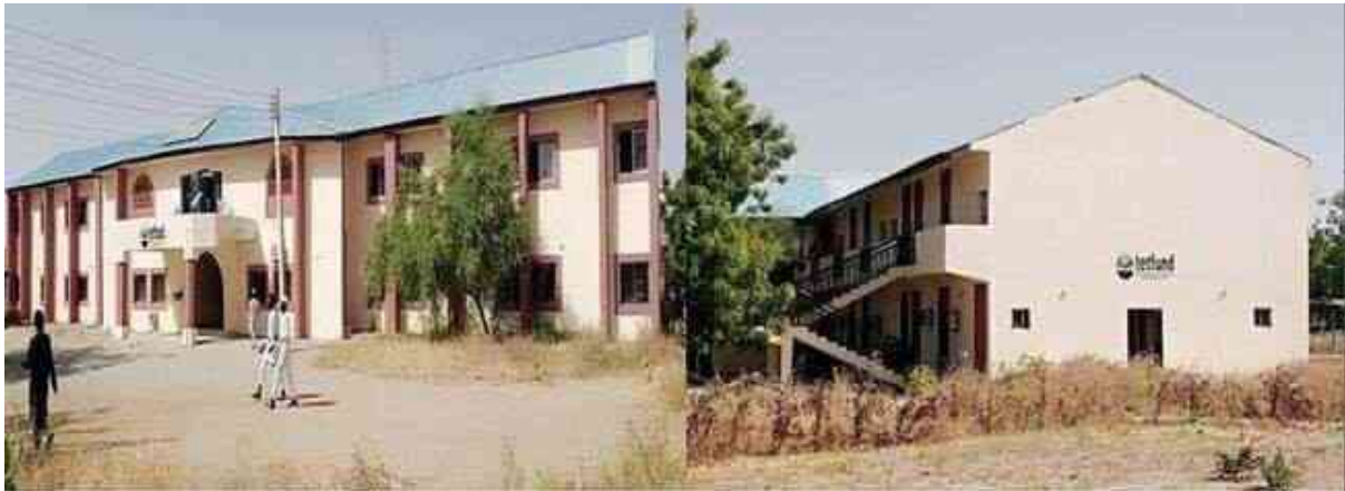
Plate 6: GNS Building – 2023 Annual Maintenance Intervention (Field Survey, 2024)
