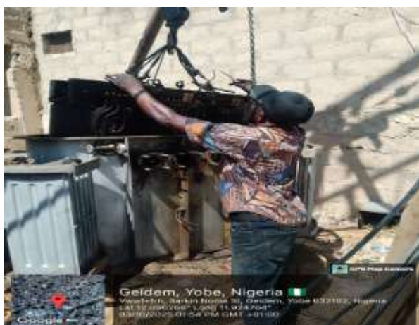
Figure 6: Corrective maintenance of 33KVA power transformer
